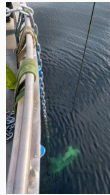
Figure 8: Anchor being lowered into water with crane.
